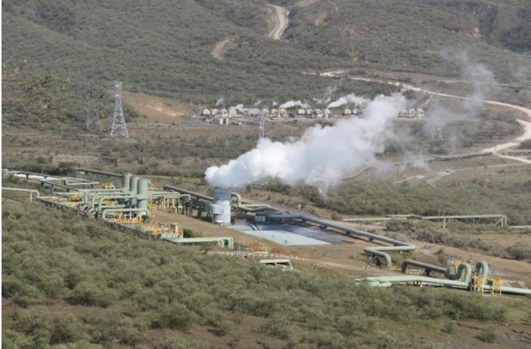
Photo: KenGen Geothermal Power Plant in Kenya (Source: Runar Magnusson, 2016)
